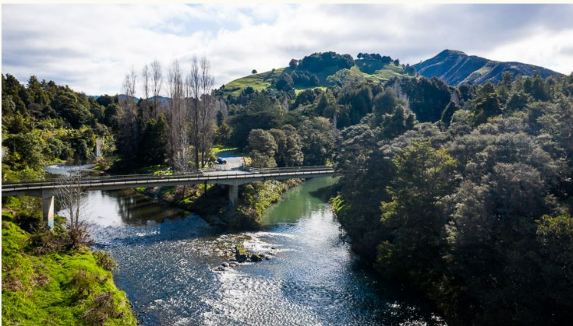
Mangakāhia River – twin bridges / Photo credit: Wendy Brown 2020
